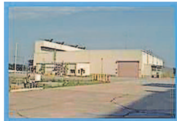
Two Glass Waste Storage Buildings at SRS will safely hold the stainless steel canisters of vitrified radioactive waste pending decisions on a permanent disposition location.
