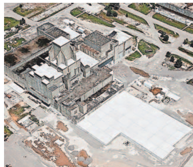
P Reactor has been permanently and safely entombed. The white concrete panels visible at the right and at various points on the building are caps covering fully grouted basins and process areas.
