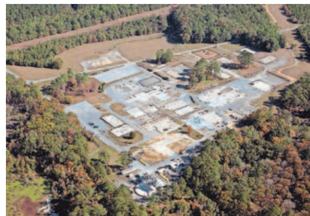
Entire areas of SRS have been closed and could be made available for future industrial uses. T Area was one of the early locations for testing various site processes and equipment, from the Defense Waste Processing Facility and high-level waste tank closure.
